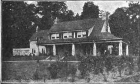
Stained with Cabot's Shingle Stains William A. Bates, architect, New York
